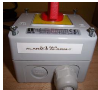
Fig. 1 Switch off contact in the Technic Box, where to the Power Supply is connected.
