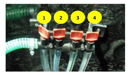
The Air Regulator must be set so that the correct volume of air is supplied to all four components inside the Vortex sewage treatment plant:
