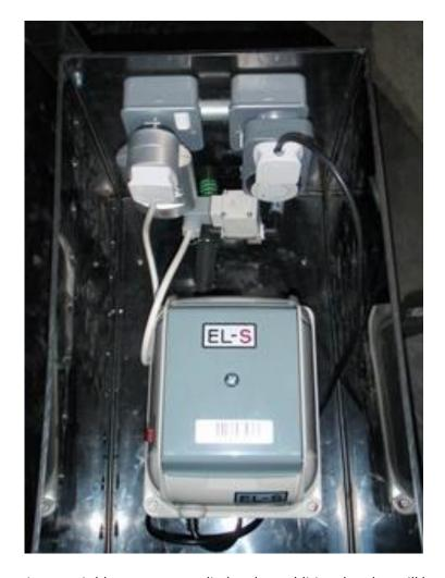
For larger Vortex units two air blowers are supplied and an additional socket will be needed.
