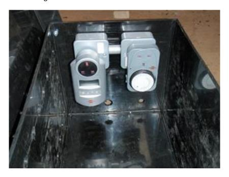
It is not possible to plug two timers into a standard double socket so for this reason multiple single sockets are required. To accommodate the timers the sockets must be spaced at least 50mm apart.
